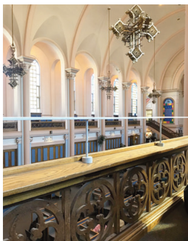
Detail of the original cast iron balustrade of the library's balconies, with the chapel light fixtures PHOTO: IRINA NAZAROVA, 2024
