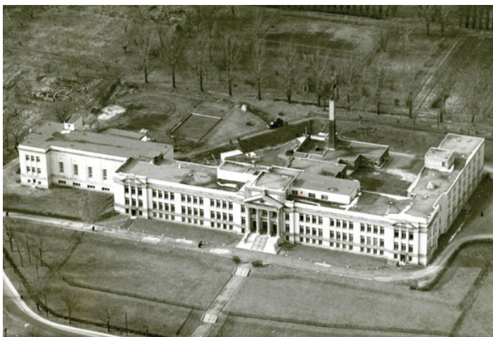
The 1950 Audet enlargement with wings on the left and right-hand sides of the central building
