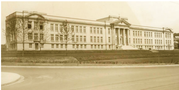
Original building at 4873 Westmount Avenue in 1926, as designed by Jean-Omer Marchand
