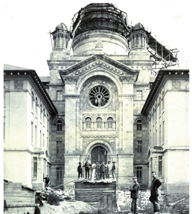
Workers at the entrance of the future 6th Mother House on Sherbrooke Street ca.1904-1908, during its construction
