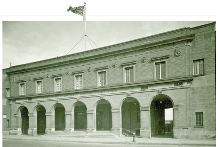
Clubhouse serving the athletic grounds of the Montreal Amateur Athletic Association, built in 1910 and located on St. Catherine Street West where Westmount High School is today.
