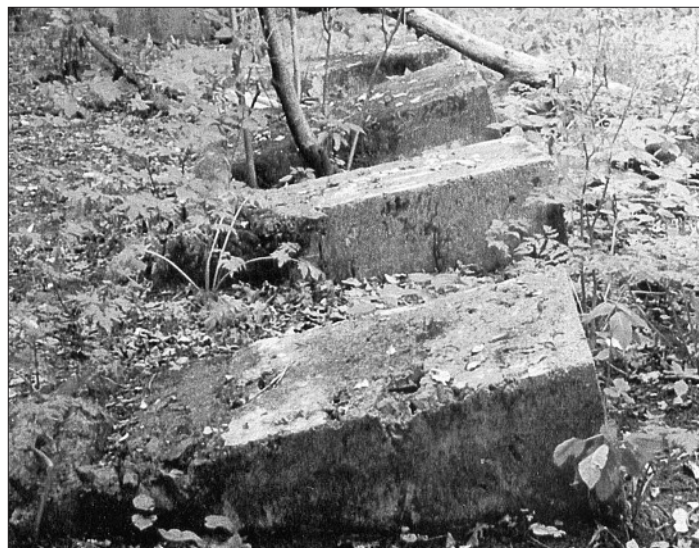
Four concrete blocks set up by the McGill Survey School in 1906 provided a base for meridian telescopes used for viewing the stars. They can still be seen today.
