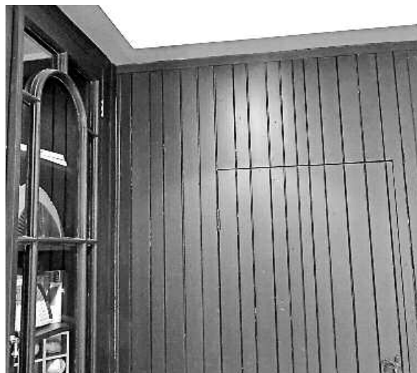
"Tongue and groove" wood panelled walls have survived since 1907 in what were originally the living quarters on the second floor for the horse's groom. The walls are now painted black and the room is used as the family study.
