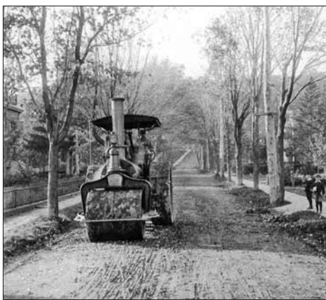
Rosemount Avenue showing preparation of road before being "macadamized"
